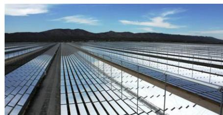
Figure 4. Linear Fresnel collector systems [9]
